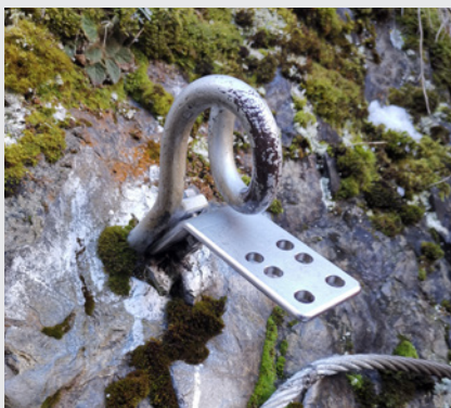
Position Ipac on the anchor in place using stainless steel bolts.
