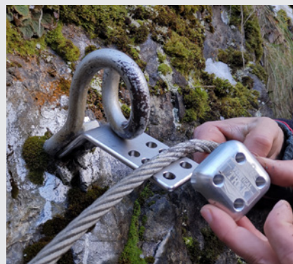
Position the die and tighten the bolts to 50 Nm.
